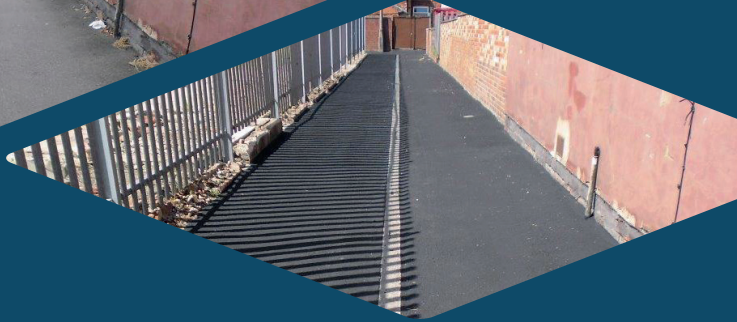
IMMEDIATELY AFTER MICROSURFACING HAS BEEN APPLIED
