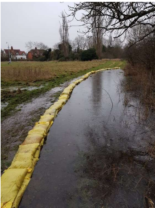
Bund along trackway
