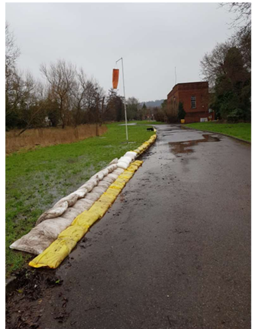
Bund on access road
